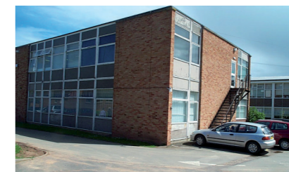
■ Chantry High School, Martley, Worcestershire Brick clad system built school
