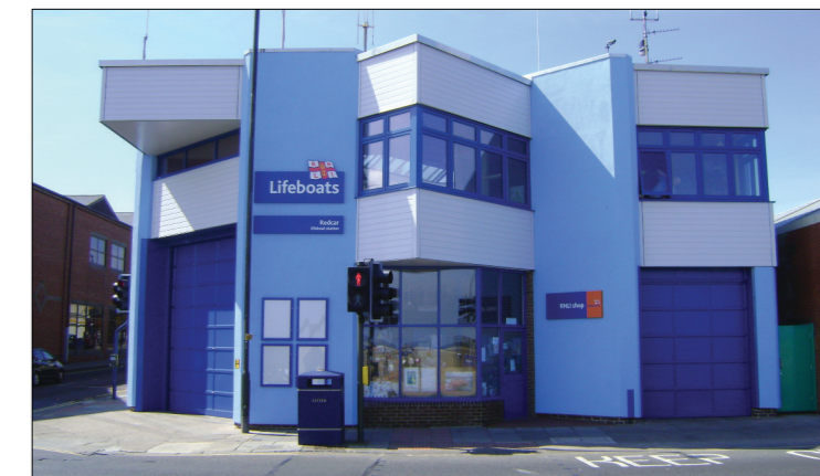
■ Redcar Lifeboat Station now benefits from an External Wall Insulation system with a silicone finish
