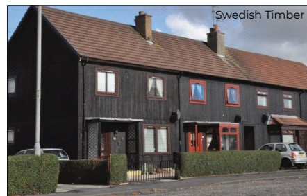
Examples of timber framed properties before refurbishment
