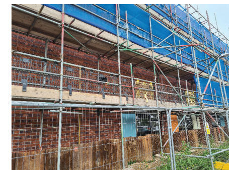
Goffs Academy during construction
