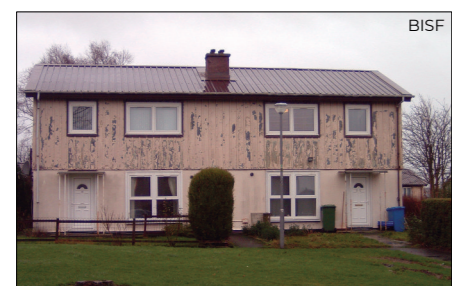
Examples of metal framed properties before refurbishment
