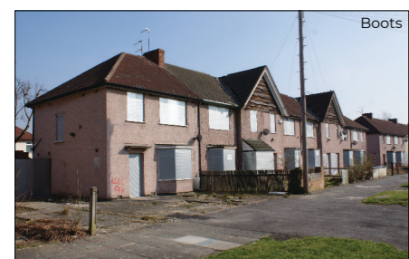
Examples of timber framed properties before refurbishment
