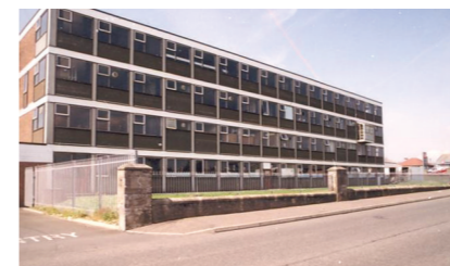
■ Ardrossan Academy, Ayrshire Concrete framed system built school
