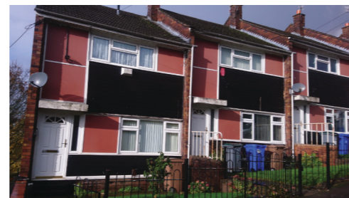
Stoke Crosswall Properties Before Refurbishment
