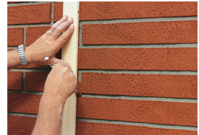
Photograph Notes: Cutting through top coat to reveal the mortar Layer.
