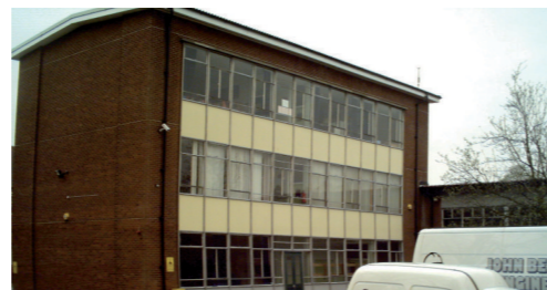
■ Kesteven & Grantham Girls School Before Refurbishment
