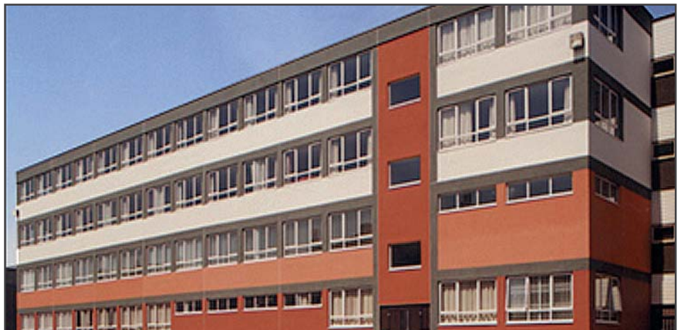
Below: After refurbishment
