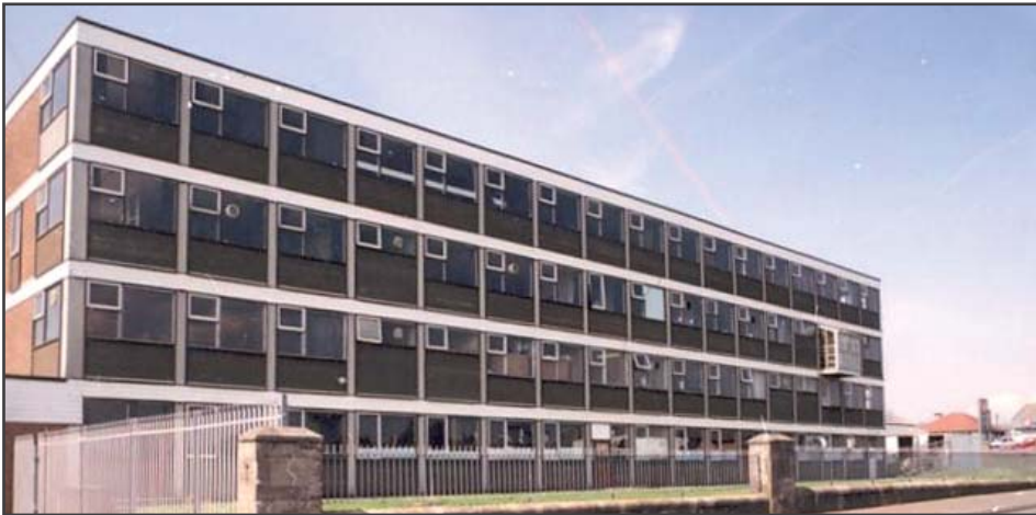
Left: Before refurbishment
