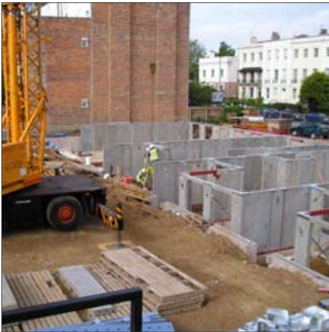
Left: Ground floor panels in situ Below: Project in progress
