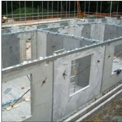
Left: Ground floor panels in place
