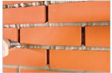
6. Pointing of mortar joint
