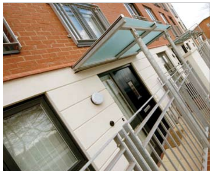
Residential Newbuild Project: High Build EWI System with Ashlar Effect Finish to Ground Floor
