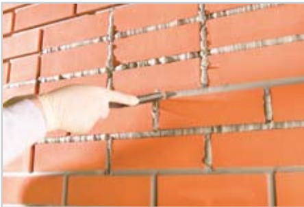
7. Tooling of the mortar joint
