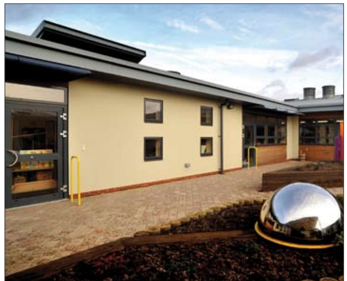
School Newbuild Project: Heavy Duty EWI System with Acrylic Finish
