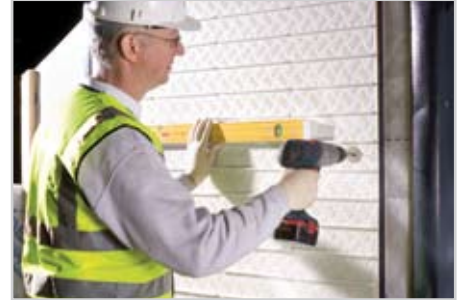
3. Attach backboard to the substrate
