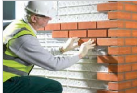
5. Adhering brick slips to backboard
