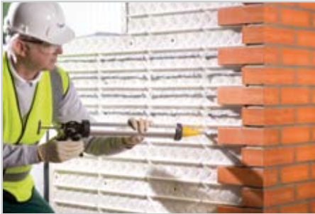
4. Application of adhesive
