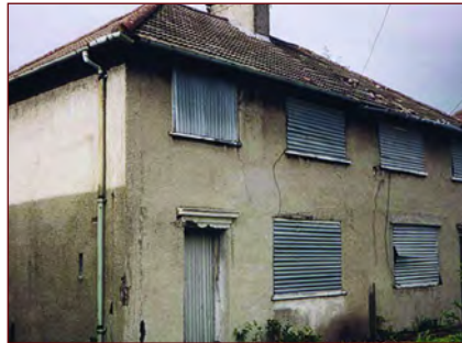
System-built housing before refurbishment
