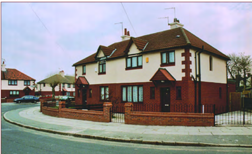
System-built housing after refurbishment
