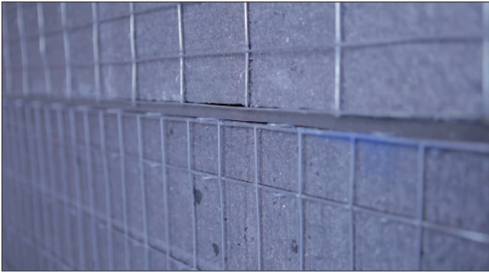
5. Before fitting the next panel the foam filler strip material should be fitted to the sides of the panels. The next panel can then be installed.
