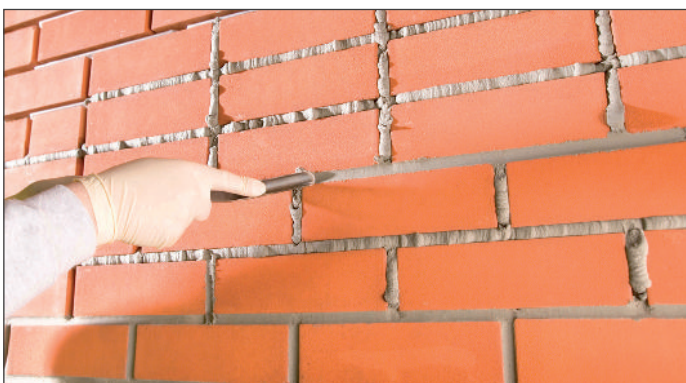
7. Tooling of the mortar joint
