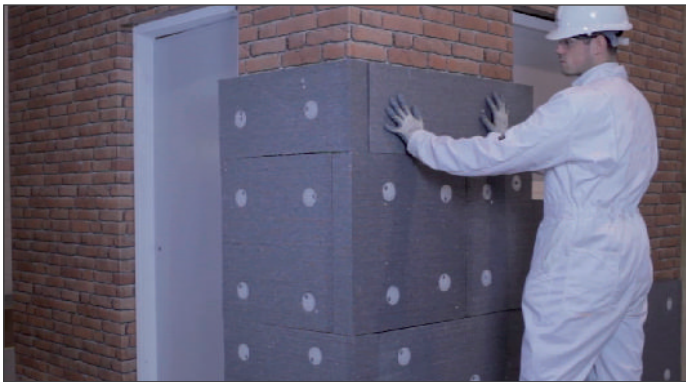
5. To ensure board above windows are 'L' shaped around windows, smaller strips maybe required.
