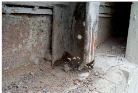
Interstitial condensation within the wall construction
