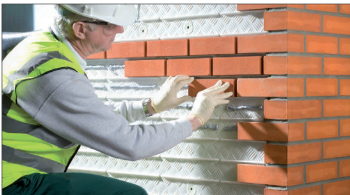
5. Adhering brick slips to carrier sheet
