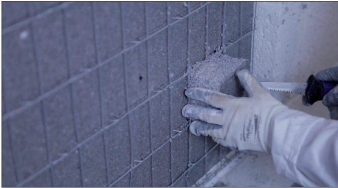
5. Remove the piece of insulation and retain for use later.
