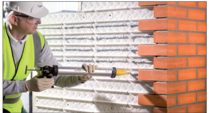
4. Application of adhesive
