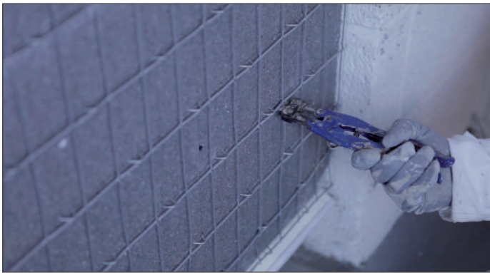
3. Measure panel and locate the fixing location on the existing building, i.e. column locations. Clip the transom wire using a wire cutter.
