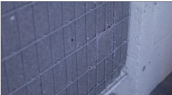
7. Replace the block of insulation back into the hole and bend the wire back to its original position.
