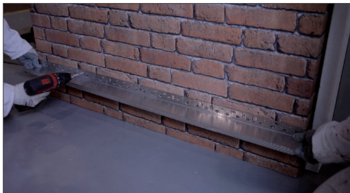
1. Install Base trim, level and fix to substrate.
