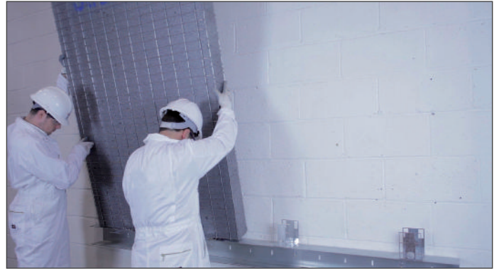
4. Insert panel into brackets, ensuring trusses line up with the brackets. The front face of the bracket can now be bent back to its original position.
