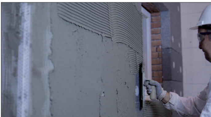
7. Apply first basecoat at 2-3mm thick using a notched trowel.
