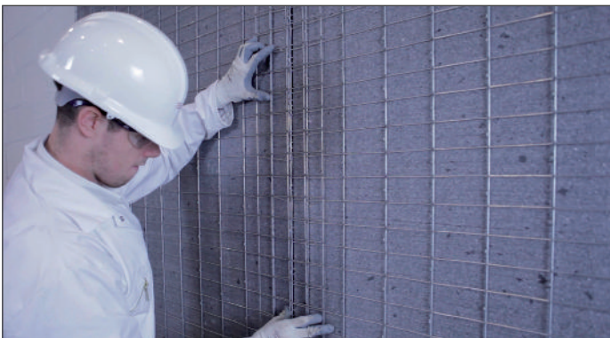
9. Before rendering can commence the panels must be fully meshed together using 200mm wide rigid flat mesh. The mesh should have a minimum overlap of 100mm and should be clipped to the truss wires of both panels using Vertex clips clamped onto the wires using a Hartco clinching tool gun (also see main photograph).
