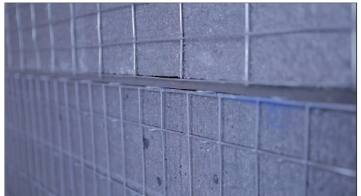
8. Before fitting the next panel the foam filler strip material should be fitted to the sides of the panels. The next panel can then be installed.
