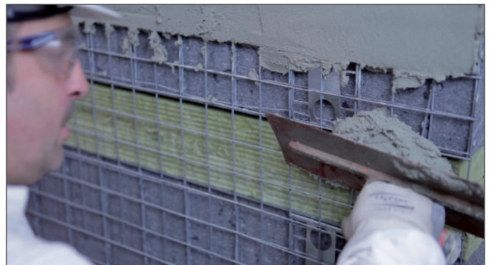
10. Basecoat render is applied in one coat 14-16mm thick. The cage must be fully covered by the render and have a minimum of 2-3mm coverage. No 'Gridding' should be seen through the first basecoat. The required finishing coats can now be applied to complete the system.
