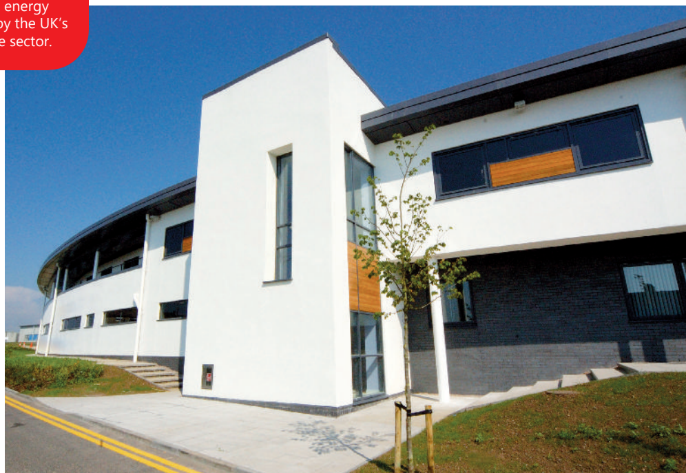
Crosshouse Maternity Unit: External Wall Insulation new build application
