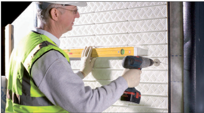
3. Attach composite panel to the substrate
