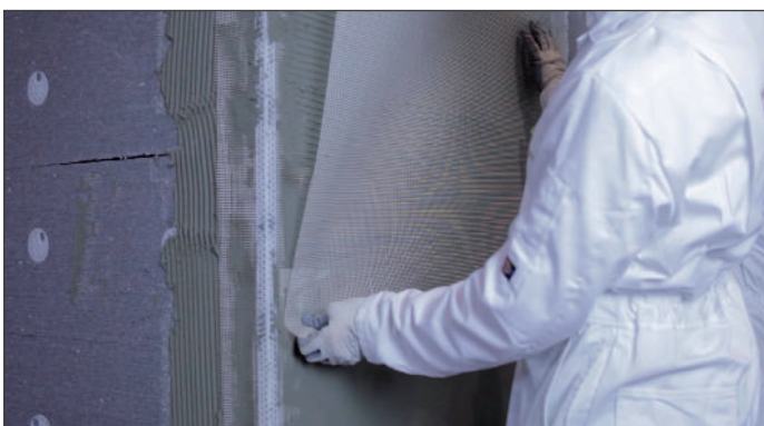
9. Ensure mesh overlaps by min 100mm at all times, including mesh on corner beads.
