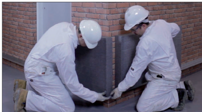
2. Locate insulation boards into base trim, ensuring correct overlap at corners.
