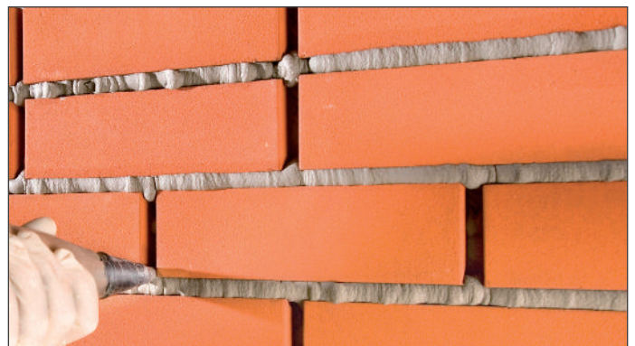
6. Pointing of mortar joint
