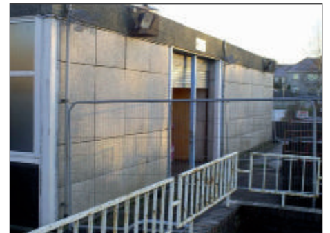
Chryston Primary School, Glasgow CLASP system built school with failing concrete cladding panels.
