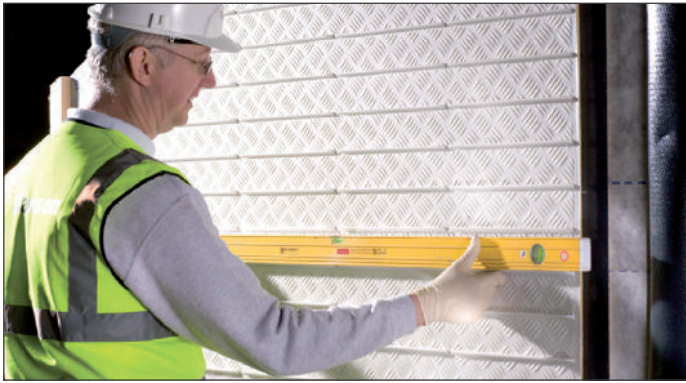
1. Alignment of composite panel
