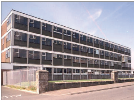
Ardrossan Academy, Ayrshire Concrete framed system built school.
