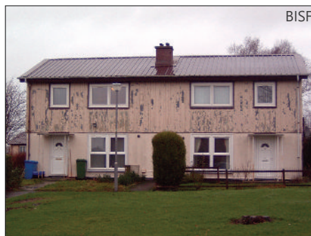
Examples of metal framed properties before refurbishment.
