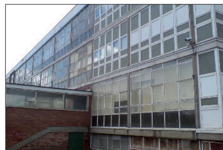
Typical system built school before refurbishment with large areas of inefficient glazing and cladding.
