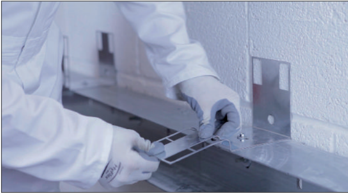
3. Bend the front face of the brackets 90°, to allow the structural panel to be inserted.
