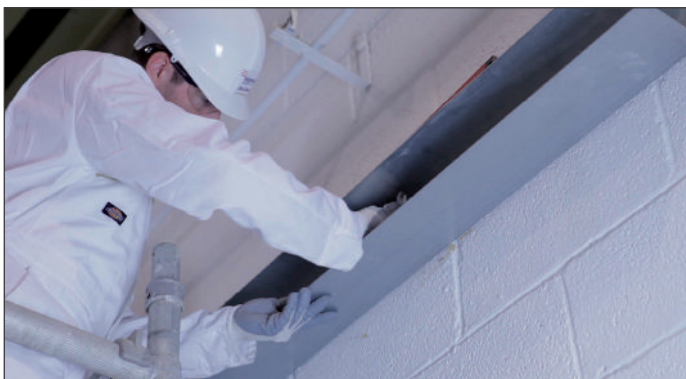
1. Install resin anchors into the floor slab or columns and then fix steel channels using washer and nut ensuring the channels are level.
