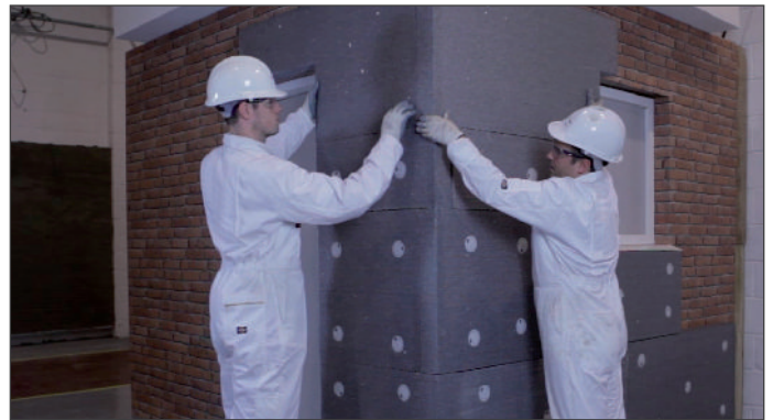
6. Cut 'L' shaped boards around window heads to reduce the risk of render cracking.
