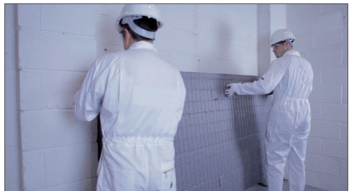
2. Panels should be cut to suit the building following the on-site panel layout diagram and then located into the base trim.
