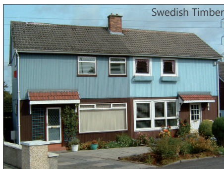
Examples of timber framed properties before refurbishment.
