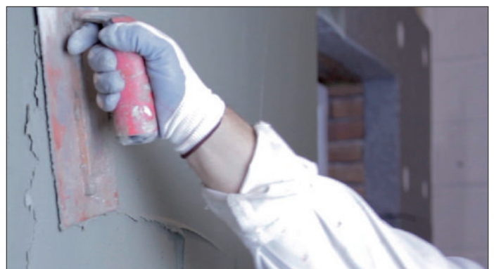
10. Apply second basecoat to a thickness of 2-3mm and smooth down with a damp sponge or float.
