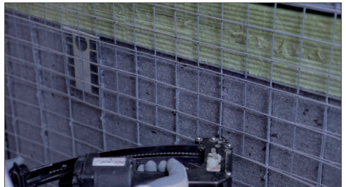
8. Rigid mesh installed over the fire break, overlapping the panels above and below by 100mm minimum, and clipped to the panels.
