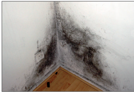
Surface condensation on the internal surface of a wall
