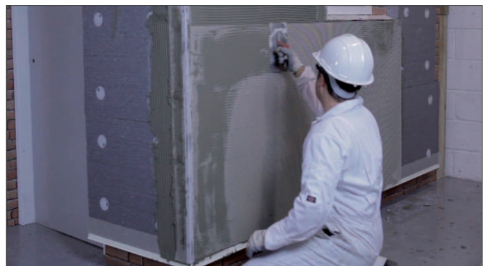
8. Bed fibre mesh into first basecoat whilst still wet.
