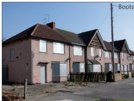
Examples of in situ concrete properties before refurbishment.
