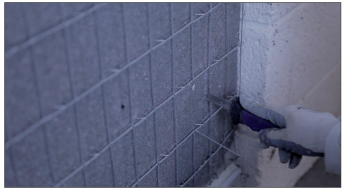
4. Bend back the cut wire and then use a pad saw to cut out a 100mm square of insulation.
