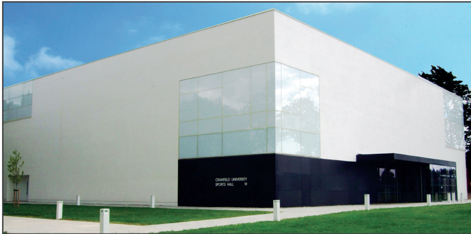
Left & Below: Large areas of render applied to create a seamless finish with no movement joints.
