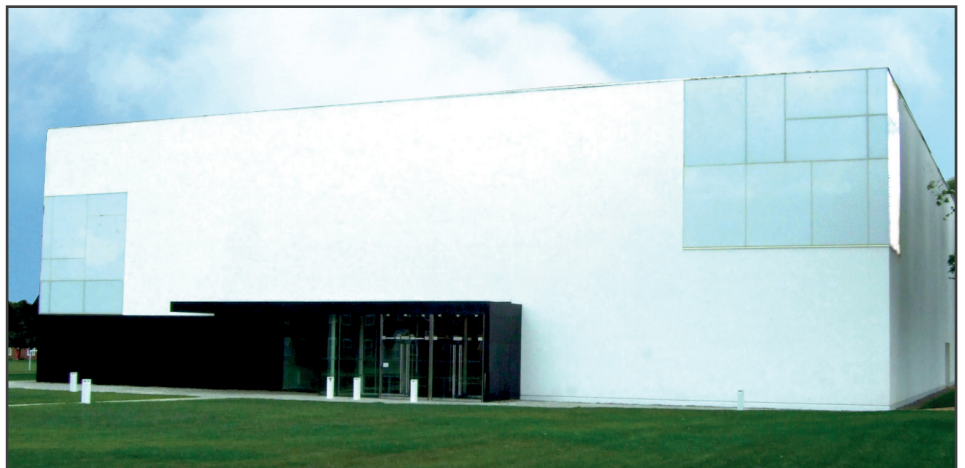
Left & Below: Large areas of render applied to create a seamless finish with no movement joints.
