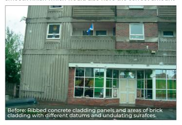
of insulation to meet stringent building regulations for thermal performance. Each elevation had six different datum levels, with the concrete edge beams protruding the furthest and the face of the brick infill recessed by 155mm (see photo bottom left). Structherm's "High Build" External Wall Insulation (EWI) was specified along with five different thicknesses of high performance Mineral Fibre insulation to overcome the different levels on each elevation.
