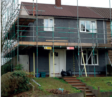
During installation of the Structural Cladding
