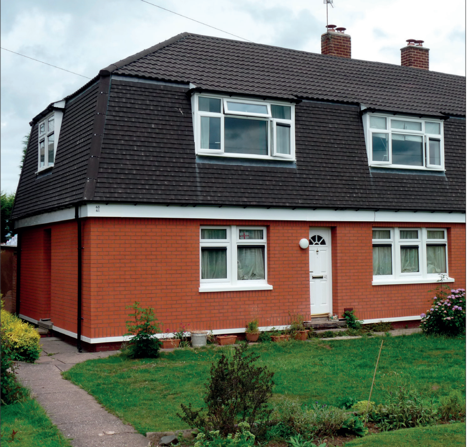
Cornish Property After Refurbishment
