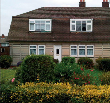
Cornish Property Before Refurbishment
