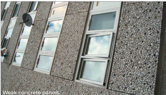
Weak concrete panels.
