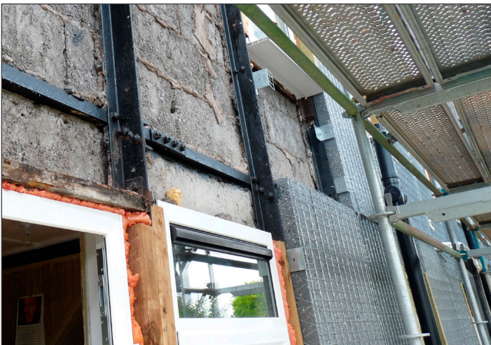
Shear receiver brackets and structural insulated cladding panels being installed between the steel columns of a stripped Dorlonco property.
