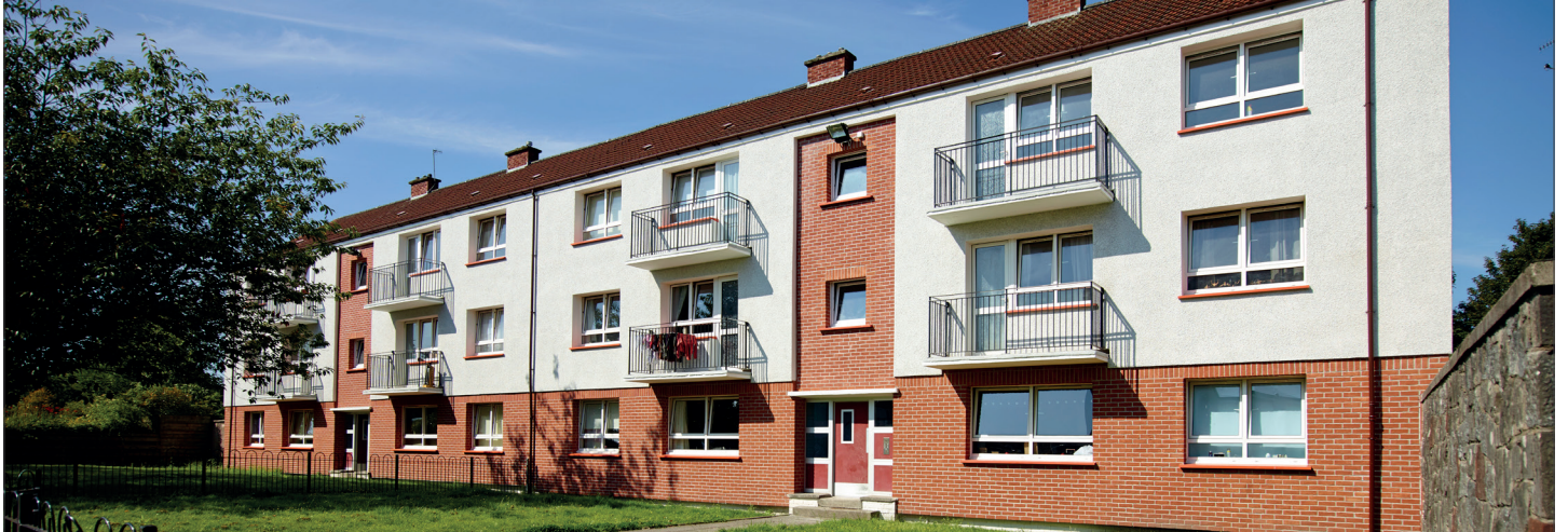
After refurbishment. Photo shows Wonderwall to ground floor and detailing areas above doorways.
