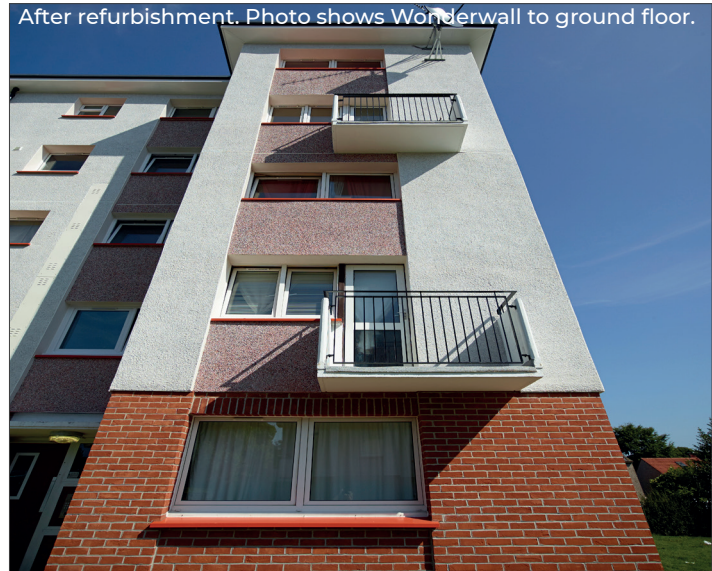
After refurbishment. Photo shows Wonderwall to ground floor.
